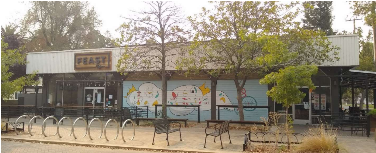
North façade, ESA 2022.
